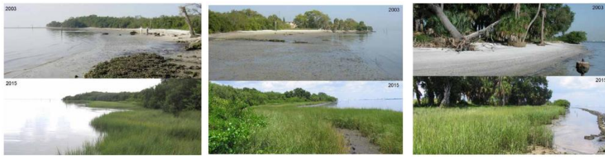
Figure 6. McDill, USAF base. Left to right: restored shoreline through the use of a nearshore oyster reef and vegetative plantings; installation of reef-building materials in the nearshore waters parallel to the shoreline resulted in the return of a highly productive and more resilient shoreline; erosion controlled with a dense vegetative buffer which resulted from the installation of a man-made oyster reef. Photo credit: Jason Kirkpatrick [13].
